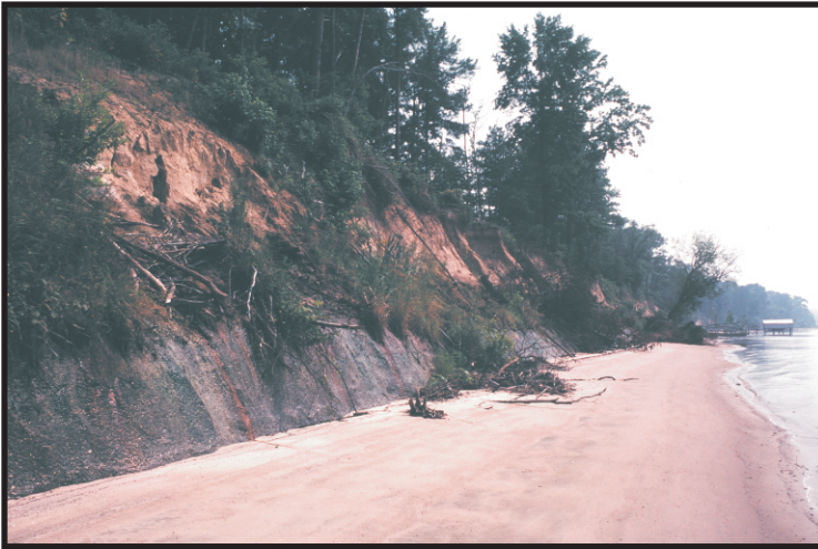
Figure 1. Exposed and eroding upland bank along the Rappahannock River, Virginia.
