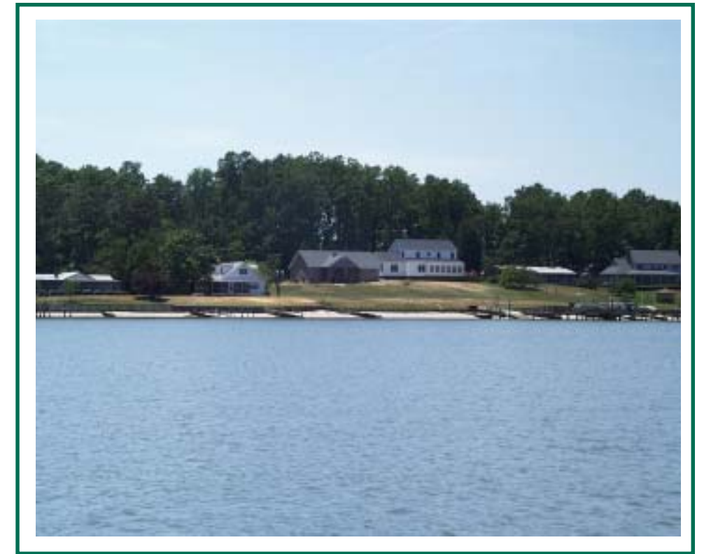
Groinfields and bulkheads along the sandy residential shore of McKans Bay.
