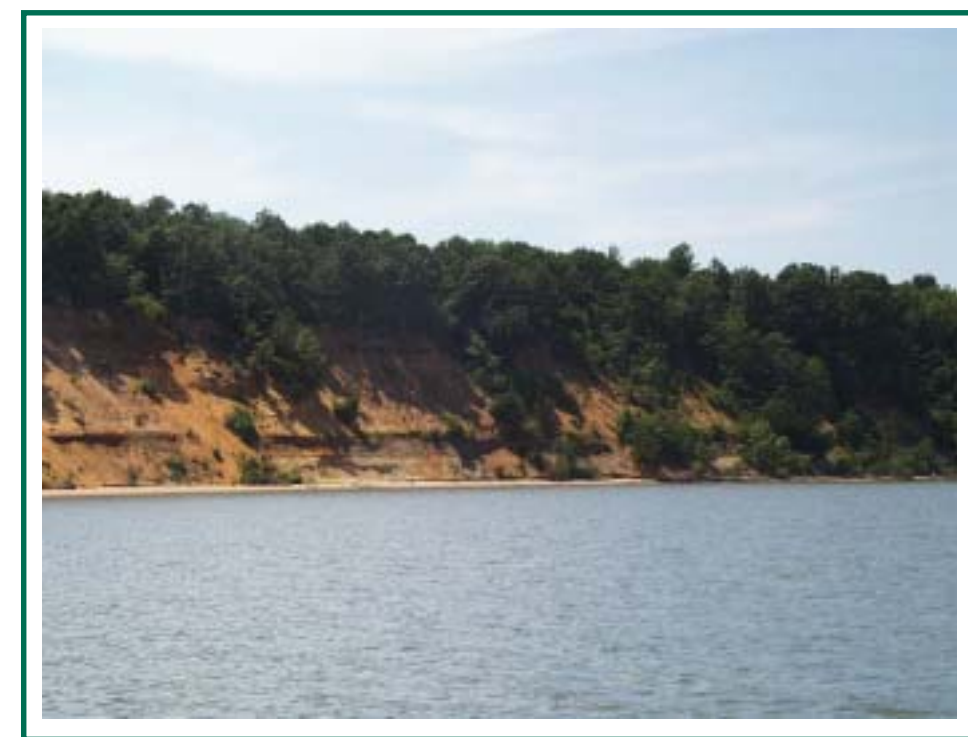
Eroding bluff along McKans Bay on the Rappahannock River.
