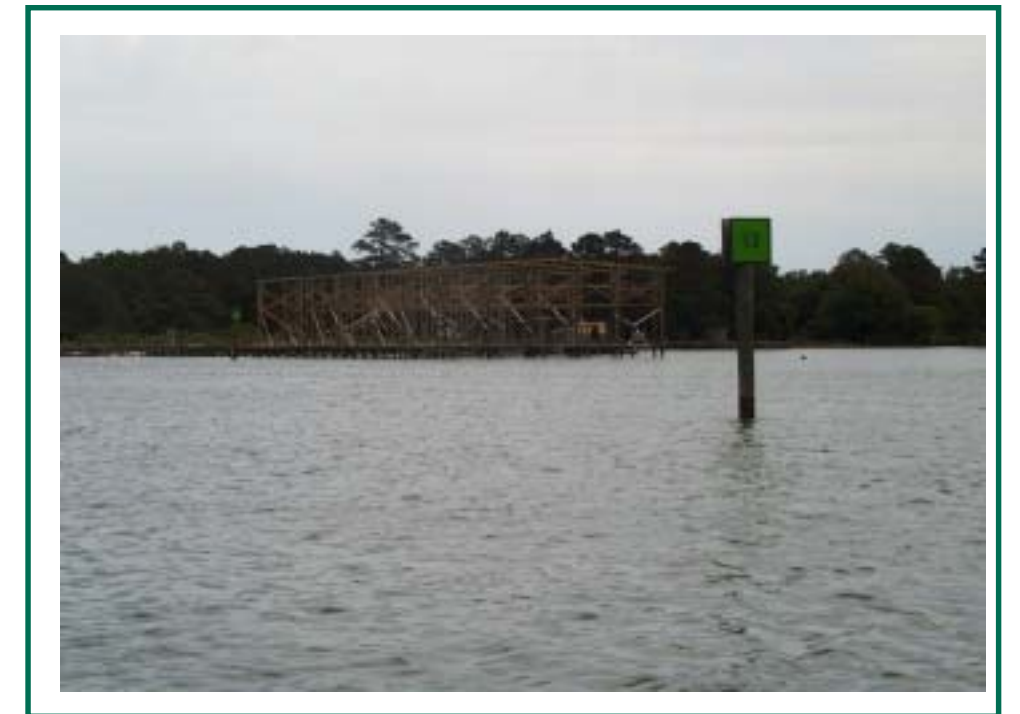
Middlesex shoreline construction.
