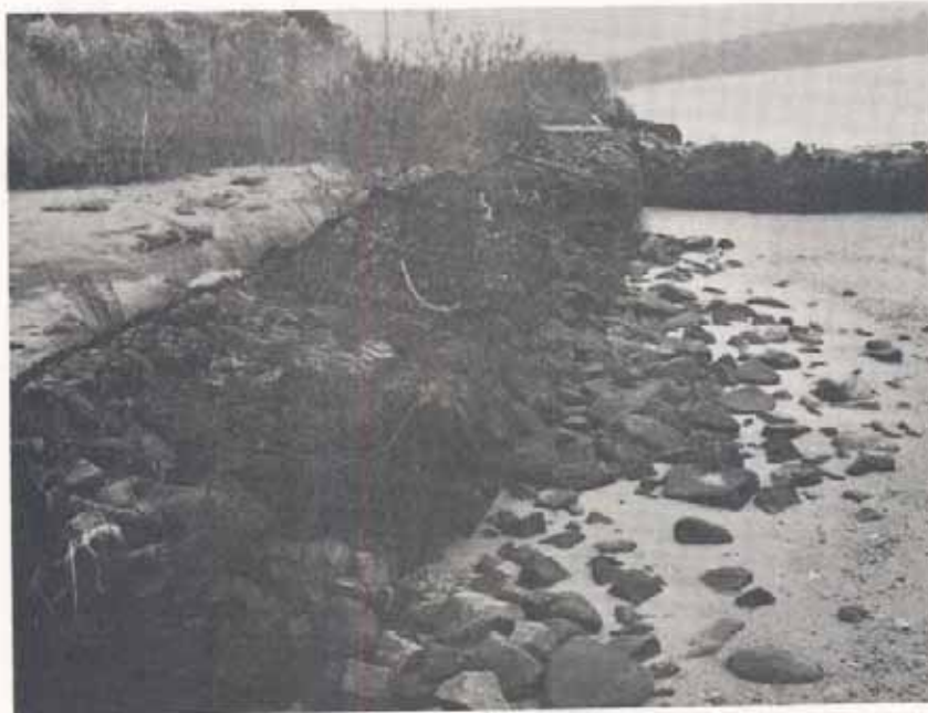
Figure ALA. West Shore Site, looking southward along the structure.
