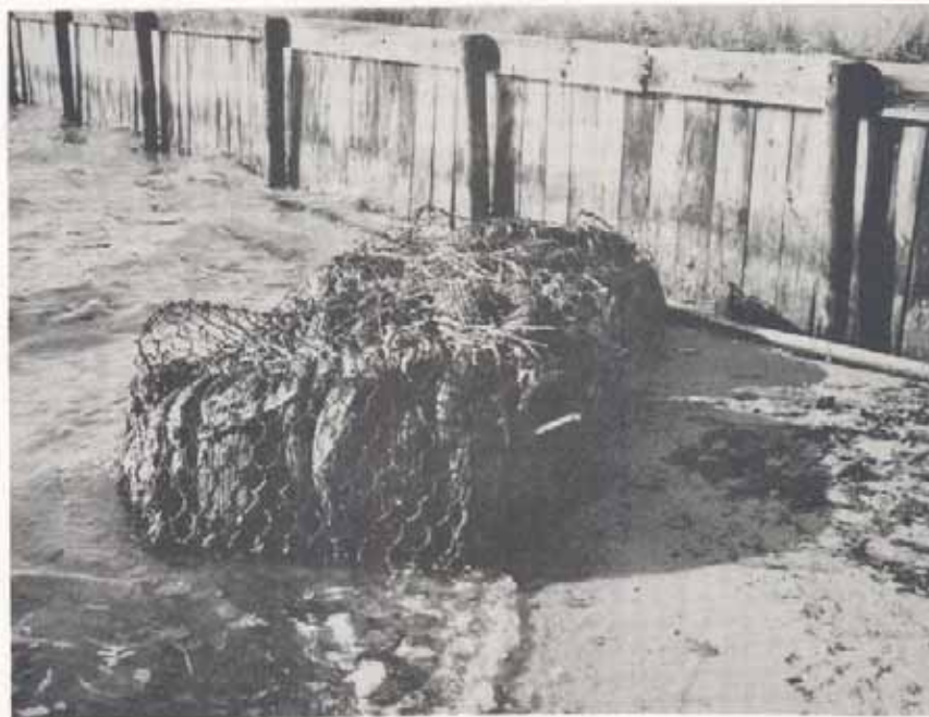
Figure A21B. VIMS Spur Site, closeup of the structure. Note tire bundles used as fill.
