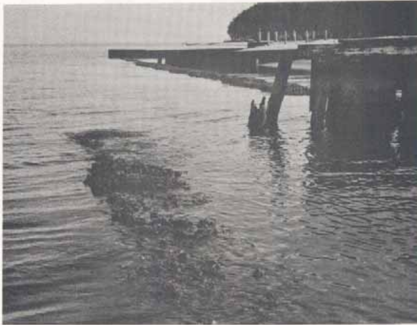
Figure AlSA. Herndon Site, looking south along sill installations 1 and 2.
