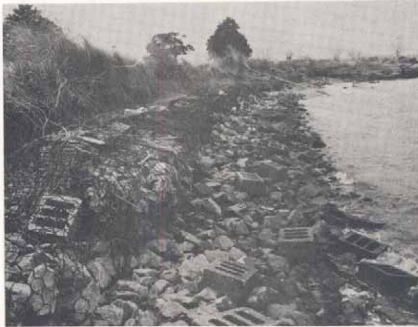
Figure A3A. Mr. Abernathy's House, looking northward along the structure.
