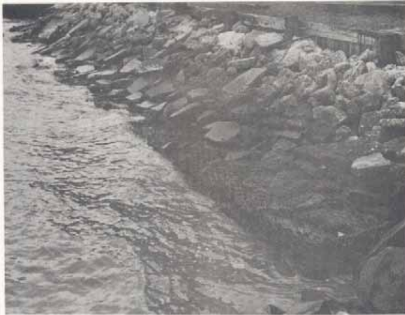
Figure AI7A. Mizelle Site, looking south along the structure.
