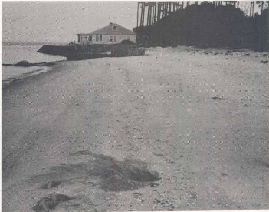
Figure A12. D. Smith Site, looking south along the shore. Sill structure is buried and runs parallel to the shore. The hole in the beach designates location of structure.
