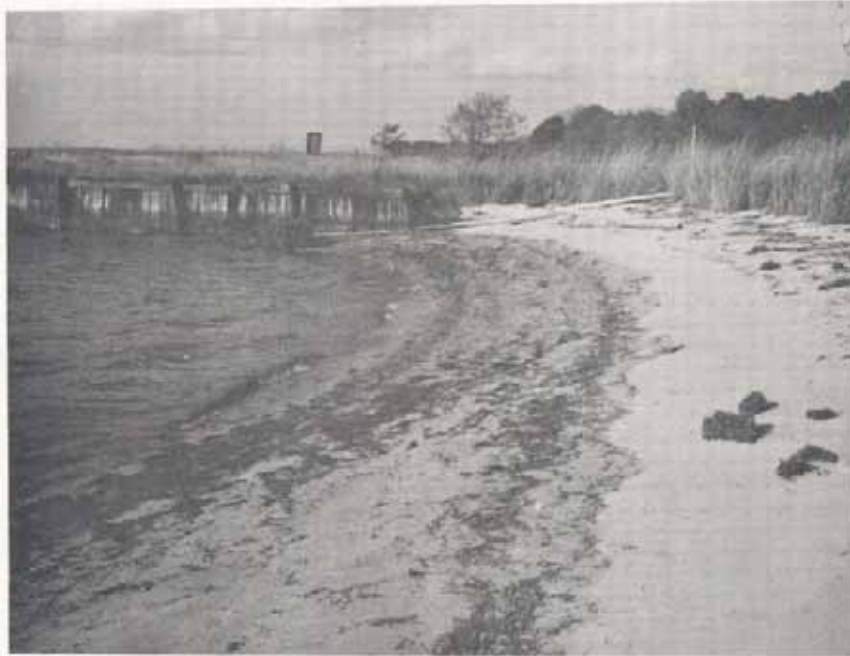
Figure A21A. VIMS Spur Site, looking north at the structure next to wooden groin.
