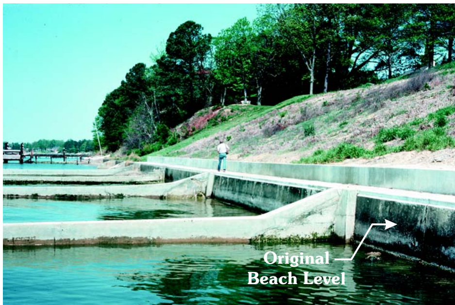
Figure 15A (top) Concrete seawall on James River in Newport News, Va.
