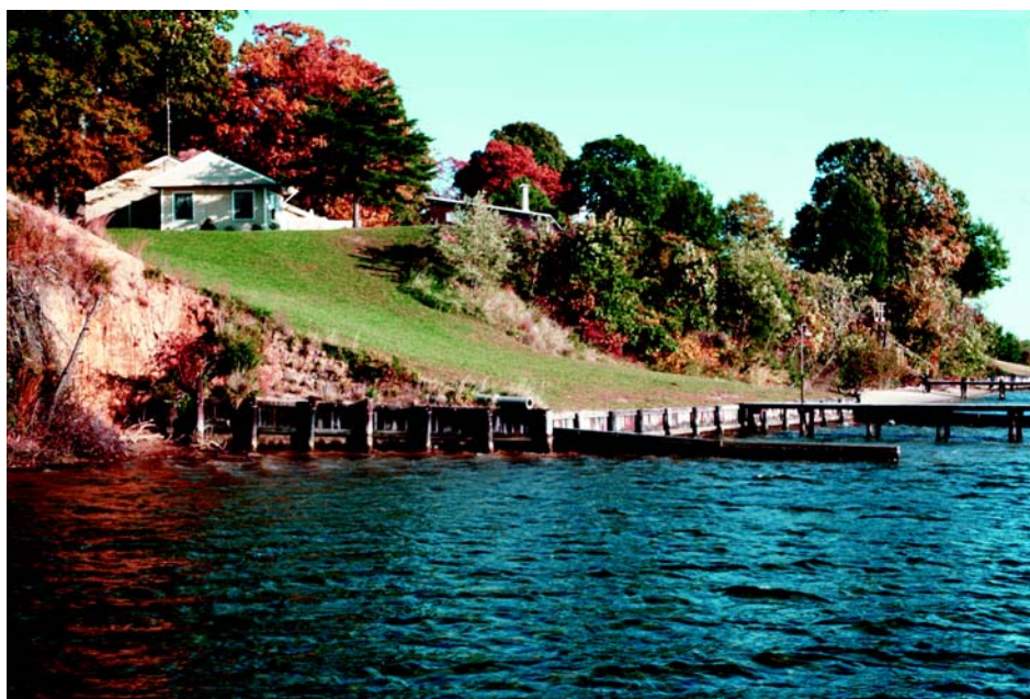
Figure 14A Bulkhead and graded bank.
