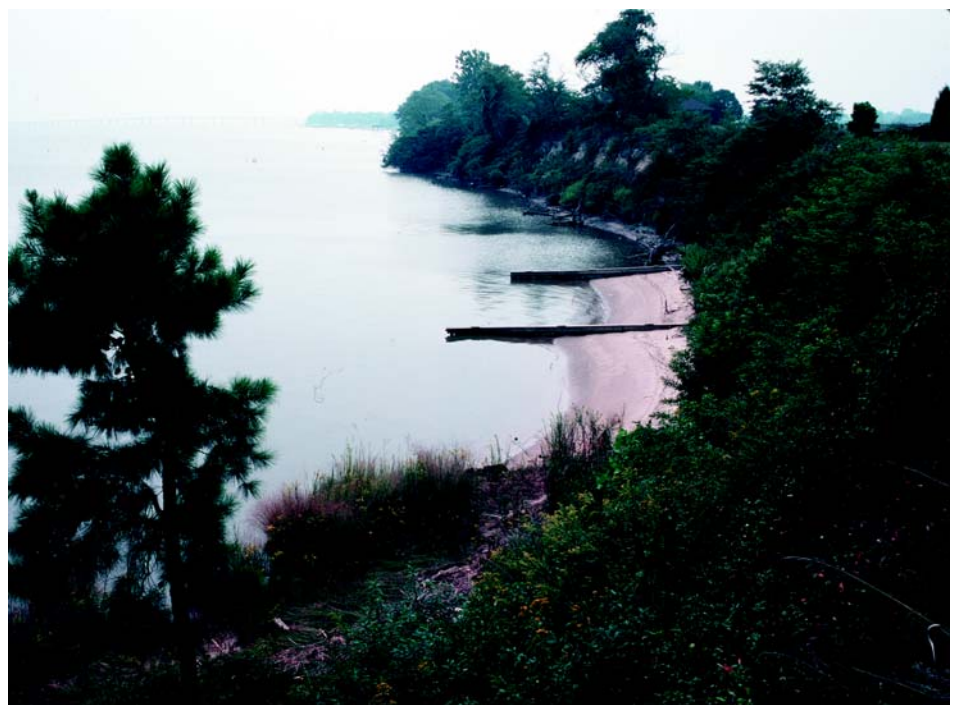
Figure 19A (top) Groin field on Rappahannock River, Va., with adequate sand supply to provide a protective beach zone to upland property.
