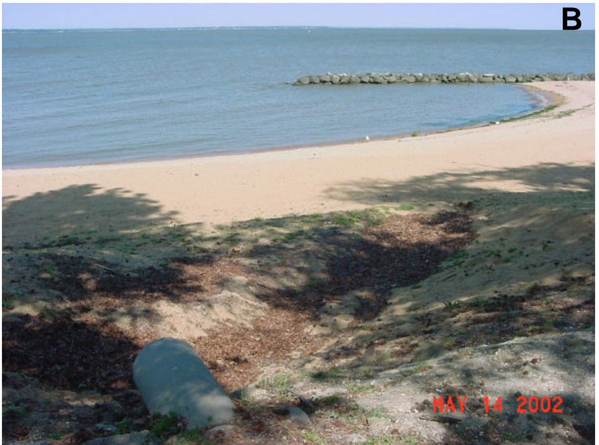
Figure 18. Central Beach storm water outfall pipe associated beach erosion A) after Hurricane Floyd in 1999 and B) in 2002.
