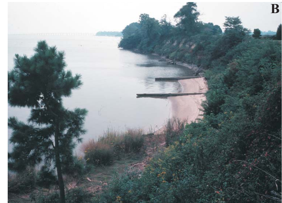
Figure 13. Groin fields A) with adequate sand supply to provide protective beach zone to upland property, and B) with an inadequate sand supply along shore reach where the topmost groin acts as a littoral barrier (from Hardaway and Byrne, 1999).
