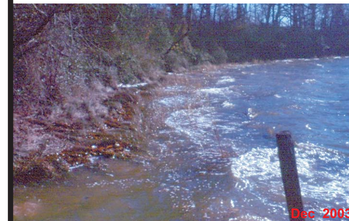
Looking south from the pier at Window 3. During a high water event with northwest winds. The water covers the sill, and the waves are attenuated by the grasses.
