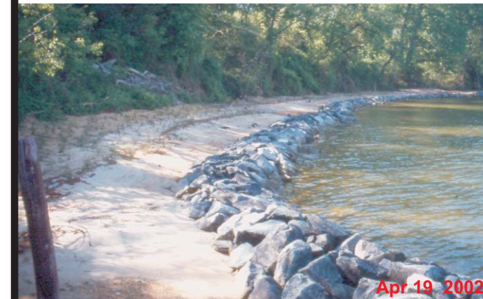
Looking south from the pier at Window 3. Spartina patens have been planted along the sand fill/terrace.
