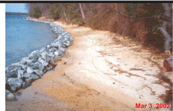
Looking north from the pier at Window 3. Post Installation.
