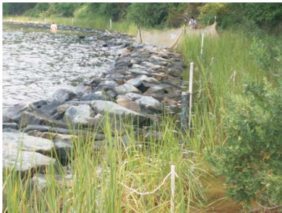
Figure 4-3. Basic sill structure with fish traps and water quality sonde in the foreground and blocking net in the background.
