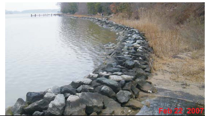
Looking north from the pier at Window 3. Five years after installation.
