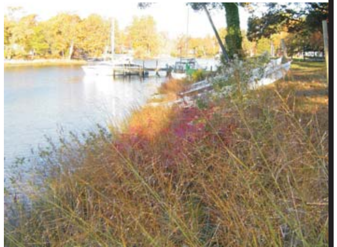
The established marsh fringe and vegetative upland slope are shown here after 24 years.
