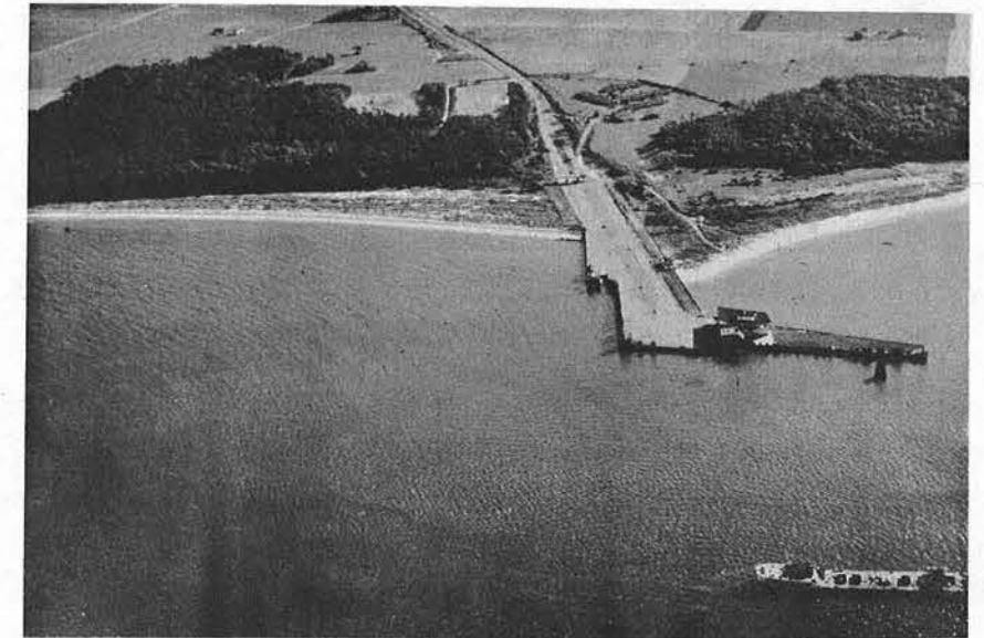
Plate 1 Kiptopeke Ferry Pier
