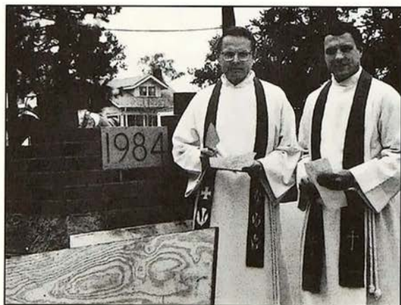
Acting President Milton Rudnick and Vice President for College Services Tom Rles presided at the cornerstone laying of Hyatt Village, November 18, 1983.
