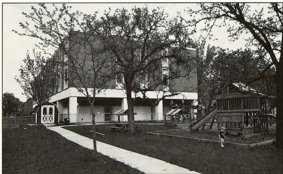
Hand-In-Hand Day Care Center occupies the first floor of Wollaeger Hall, and has a well-equipped play area adjacent to it.
