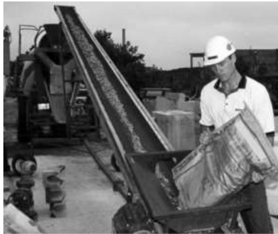
Figure 2.12 Adding fibres last to the transit mixer [76]
