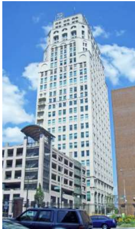
Figure 2.3 Southwestern Bell Telephone Office (Oak Tower) [11]
