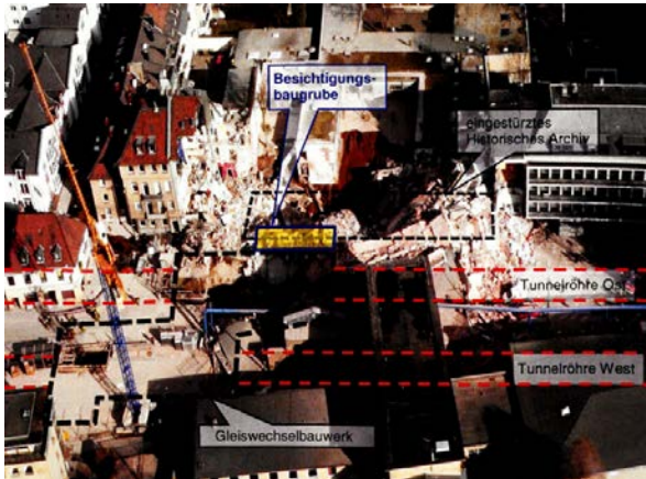
(a) Failure of the historical archive (Moormann et al. 2014)
