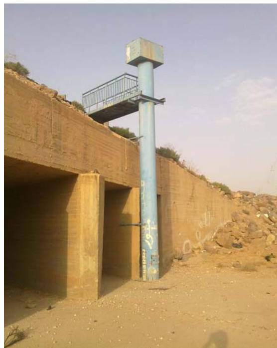
Figure 7. Al-Za'atari gauging station including chart recorder (Stevens Type A)
