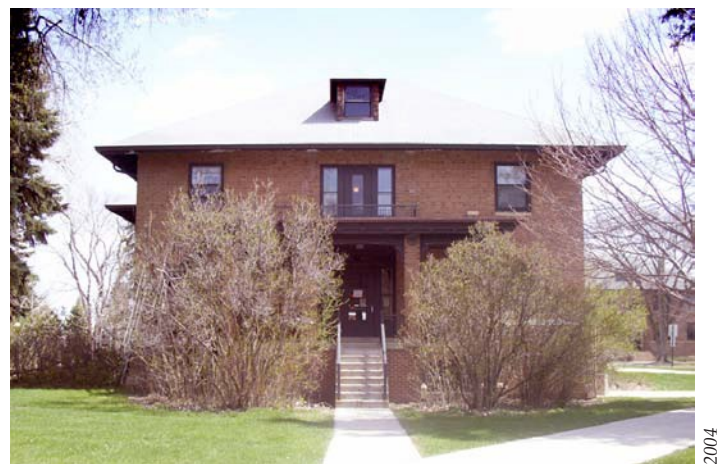
West Elevation: This elevation faces the Humanities Building.
