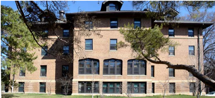
South Elevation: This elevation faces Miller Field and Gay Hall.
