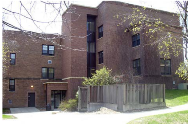
Behmler Hall's 1980s elevator tower addition is tucked into a rear corner. The addition's footprint is minimal and its materials and detailing are compatible.
