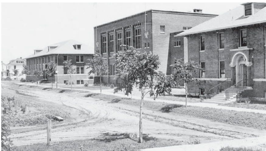
Behmler Hall flanked by Social Science and Blakely Hall. Note Blakely's original main entrance. The building at the left edge is a herdsman's house.
