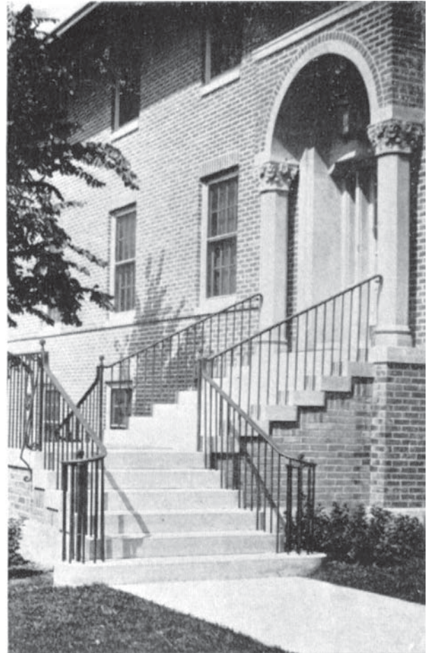
Pine Hall's main entrance with double stairway and stone columns was removed in 1968.
