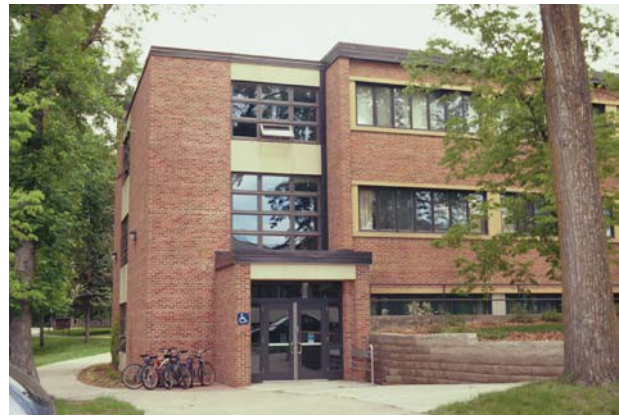
This successful 1997 stair and elevator addition on Humanities is placed on a side wall away from the historic main entrance, is well-scaled, and has compatible materials and detailing.
