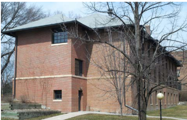
South Elevation: This elevation faces Gay Hall.
