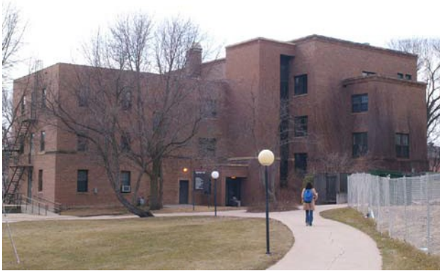
North Elevation: This elevation faces the Social Science Building.
