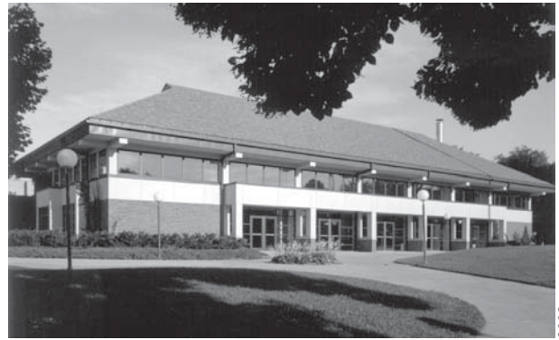
The building's 1992 expansion has a hipped roof to complement the historic buildings around the Mall.
