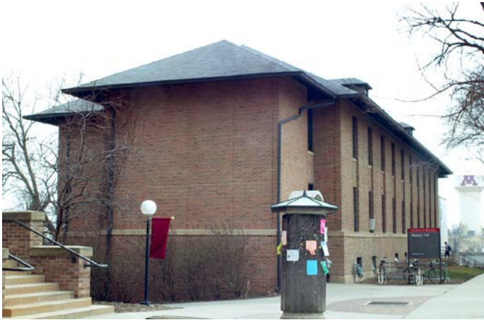
North Elevation: This elevation faces Behmler Hall.
