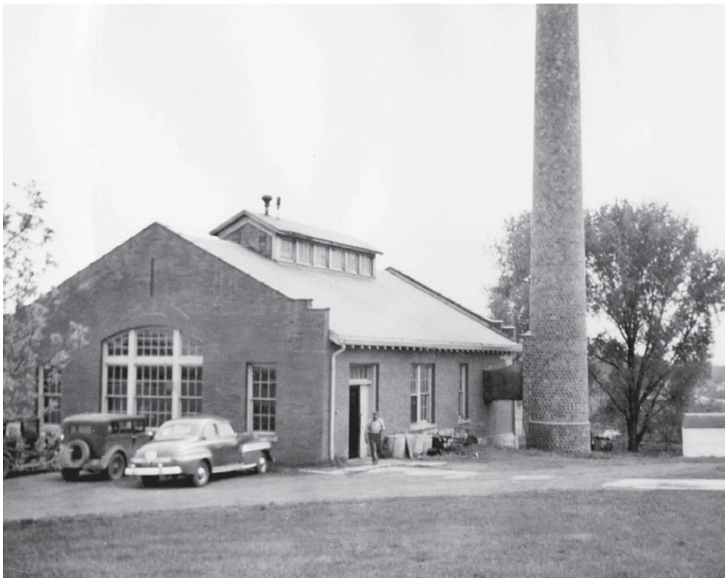
WCSA heating plant east of Behmler Hall (razed).
