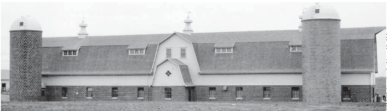
At 175 feet long, the Cattle Barn is an impressive structure. Silos on the west façade (now gone) were built of hollow tile, brick, and later glass-lined steel. The roof was rebuilt after the 1950 hay mow fire.
