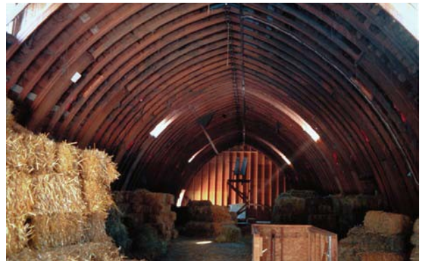
Exposed laminated wood rafters in the Saddle Club Barn.
