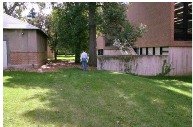
Narrow linear space between HFA and the two courts. Note the cast-in-place concrete retaining wall that serves to draw HFA's modern-era materials into the space.
