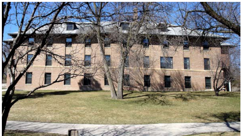
East Elevation: This elevation faces the Food Service building.
