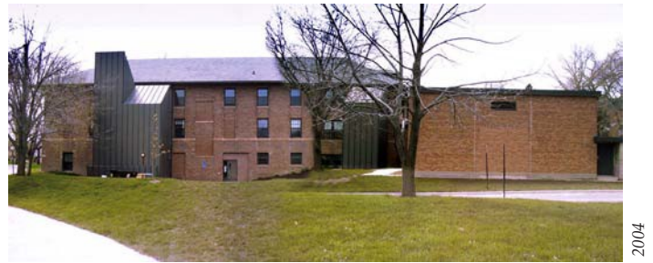
East Elevation: This elevation faces the residential halls zone. (Photo predates recent rehabilitation.)
