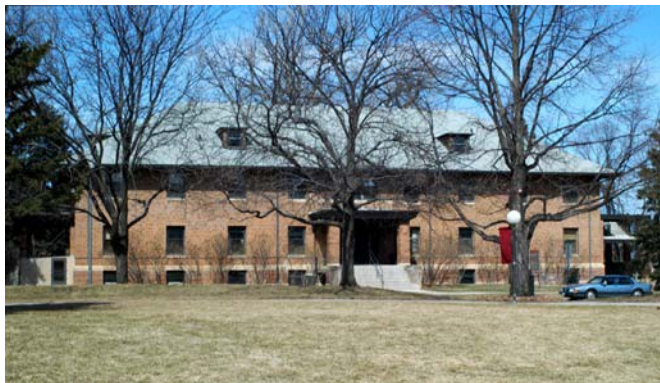
South Elevation: This elevation faces the Mall.
