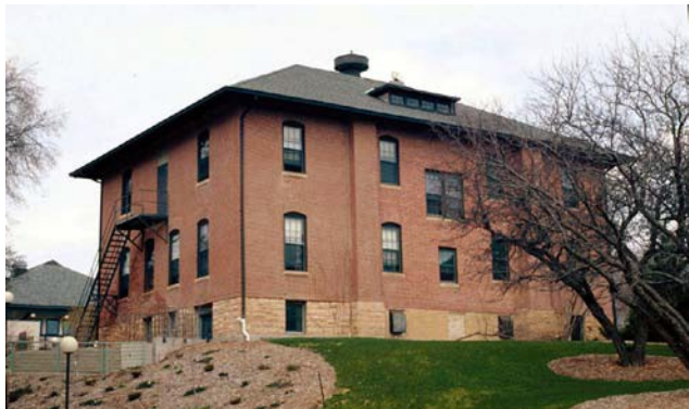
South Elevation: This elevation faces Miller Field.
