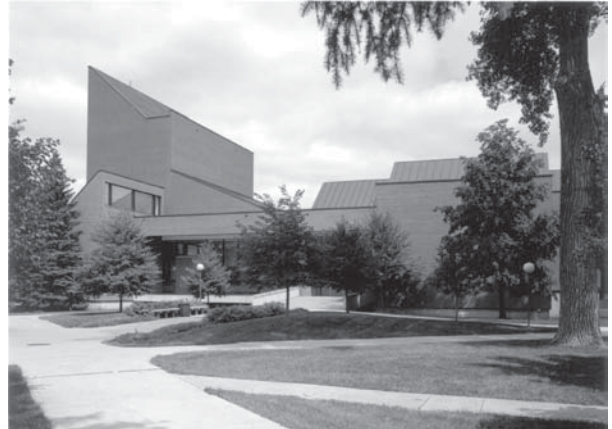
HFA's towers are roofed with standing-seam coated metal. The building was designed by Ralph Rapson and completed in 1973.
