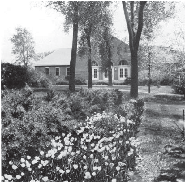
The WCSA's original Administration Building looked north into the Pine Hall Glen. This circa 1932 view shows the open areas of sunlight and tulip beds that existed just north of Cougar Circle.
