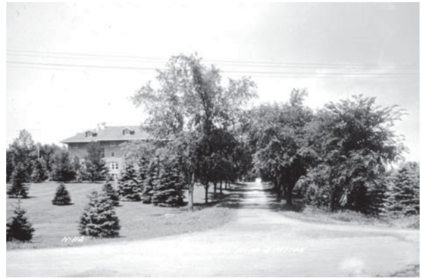
The south end of the north-south road, taken from Second Street.
