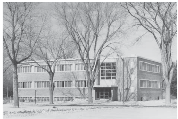
Humanities was designed by Bernard J. Hein who also designed Edson Hall, the Social Science north addition, and other work on campus.
