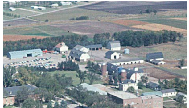
The farm buildings were arranged orthogonally and oriented to the campus grid.
