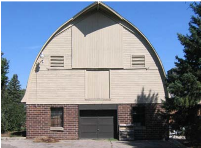
South Elevation: This elevation faces Social Science and the lawn west of the residential apartments.
