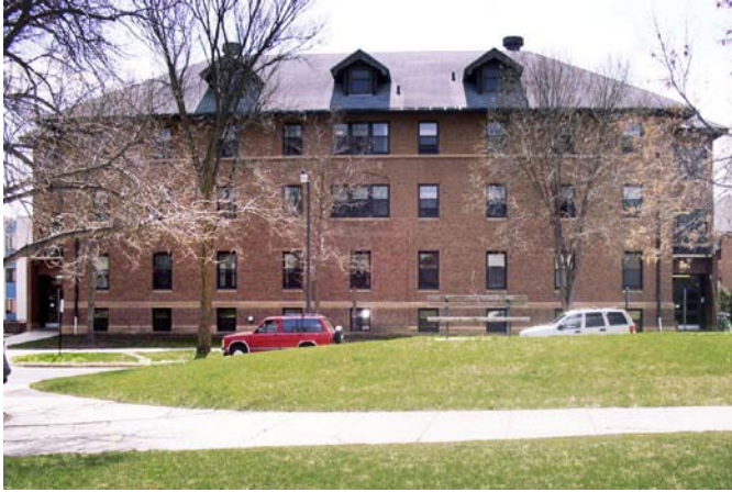
North Elevation: This elevation faces the Mall.
