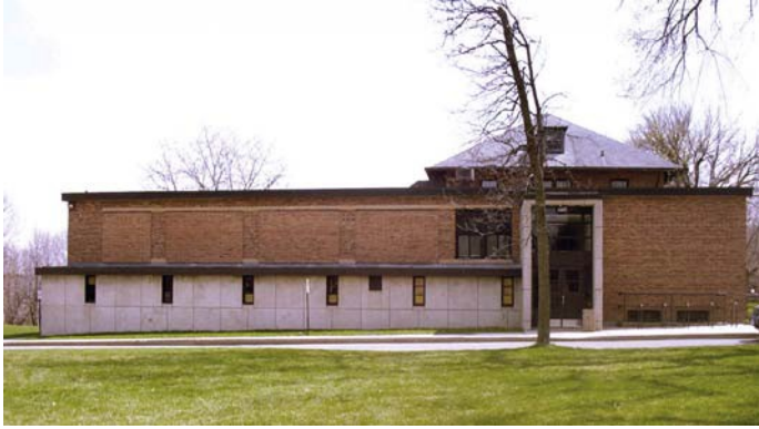
North Elevation: This elevation faces the lawn west of the Saddle Club Barn. (Photo predates recent rehabilitation.)
