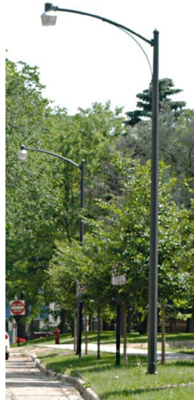
The “University Standard” streetlight was first used on campus circa 1955. It is recommended that these poles be retained.
