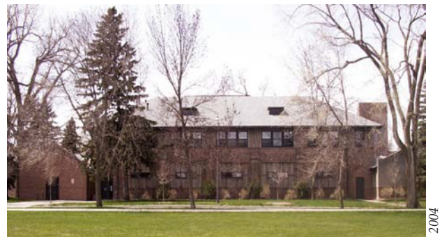
East Elevation: This elevation faces the lawn west of the Saddle Club Barn.
