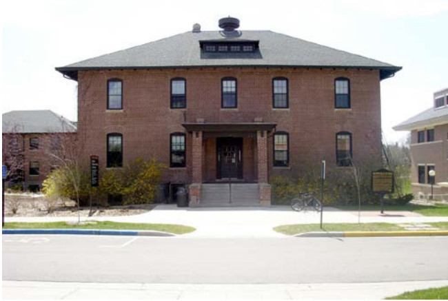
North Elevation: This elevation faces the Mall and the Student Center.
