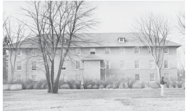
Pine Hall's 1968 stair tower addition was insensitively placed in the center of the main façade, replacing the historic main entrance.
