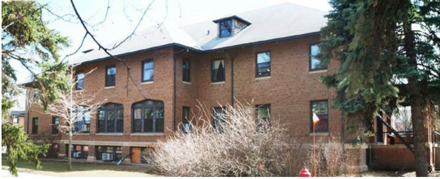
North Elevation: This elevation faces the Community Services Building.
