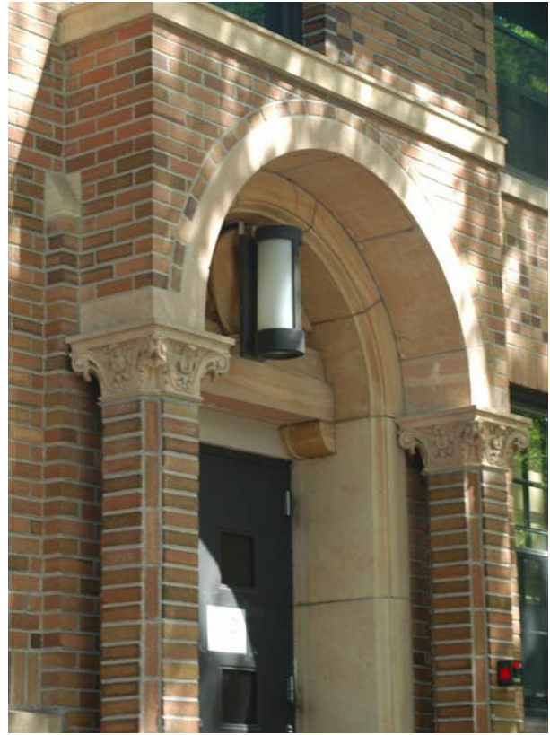
Brick columns and Kasota stone mark the main entrance to Social Science.
