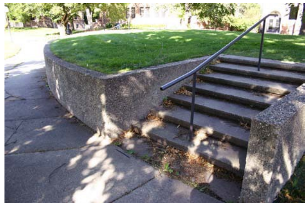
The stage is integral to the 1968 Roger Martin design. The texture of the aggregate concrete, the scale of the shallow, recessed steps and the gentle angle of the metal rail create an elegant minimalist expression of late 1960s American landscape architecture.
