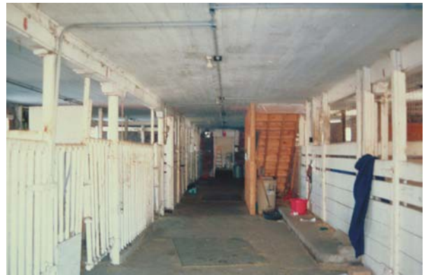
The wood ceiling patterns, stalls and posts of the barn interior are a unique legacy of the WCSA era.
