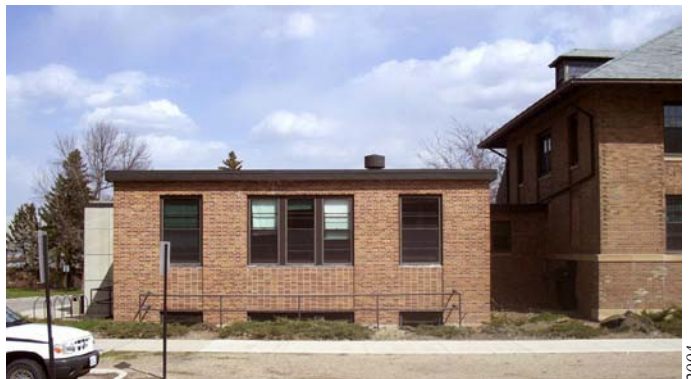
The 1950 north addition to Social Science was set apart from the original building in a way that allowed the 1920 massing and design to continue to be conveyed. (This addition is being altered in the Social Science rehabilitation project.)
