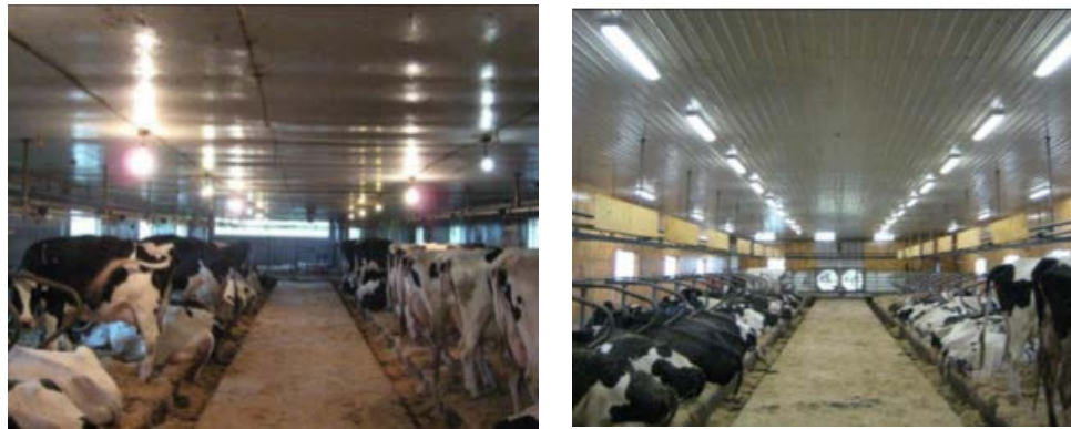
Figure 2: Left: A dairy barn with incandescent lighting. Right: A dairy barn with LED high efficiency lighting (Carrie Houston, et.al, 2013).
