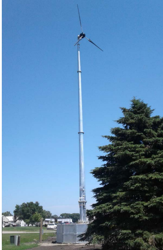
Figure 7: One of the two 10 kW Ventera wind turbines installed at the WCROC dairy farm.
