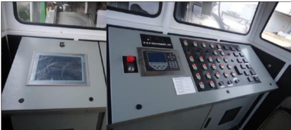
Figure 5. RAR Production Plant. (After (33))
