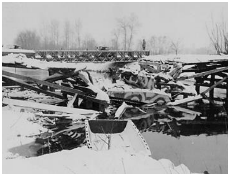
Figure 6. The collapsed bridge and tank at the Ill River crossing.
