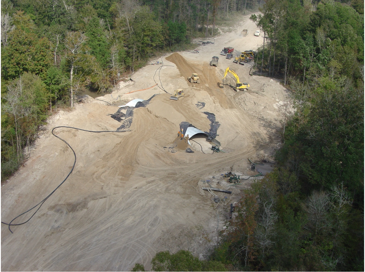
Figure A3. DMPBAC culvert
