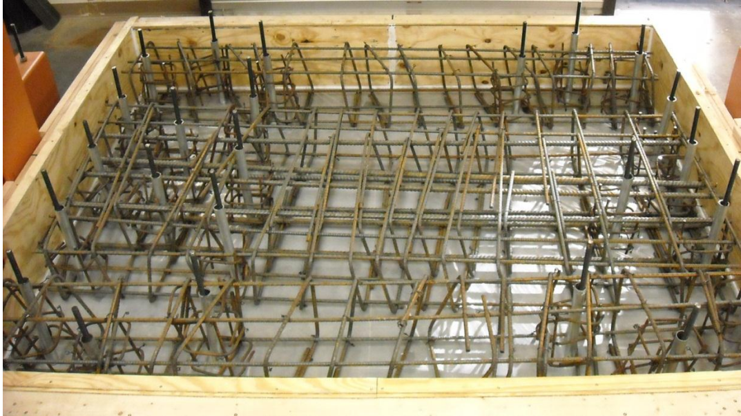
Figure 5.3: Foundation Rebar: Rebar Cages Arranged in Foundation
