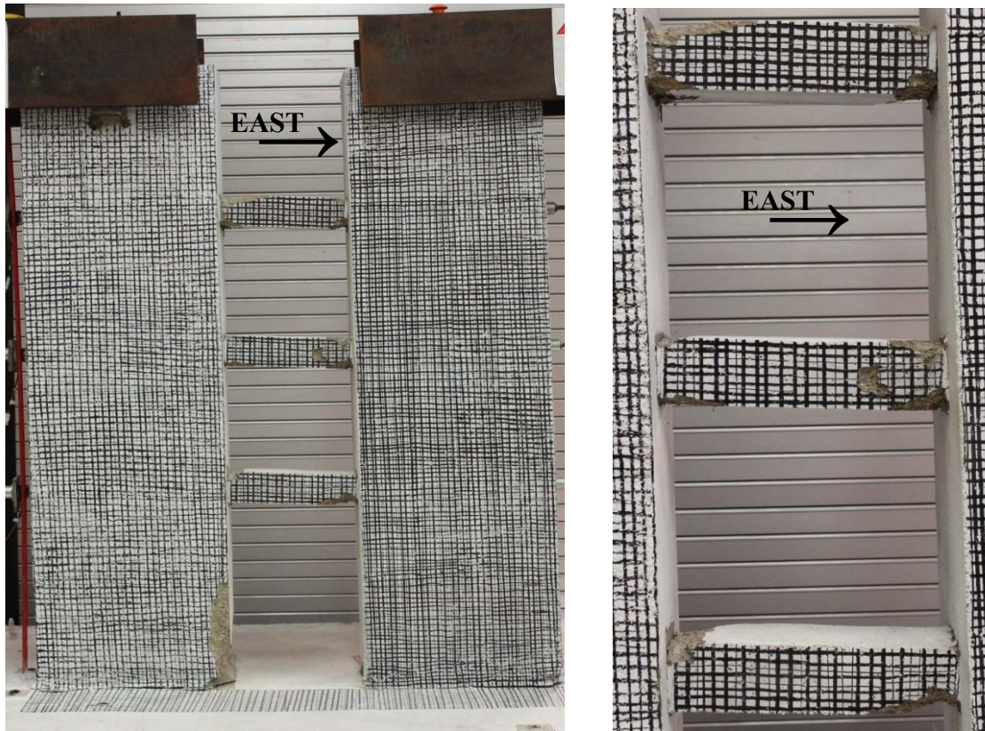
Figure 7.60: Specimen Damage After Testing (Looking North): (a) Global FOV; (b) Beam
