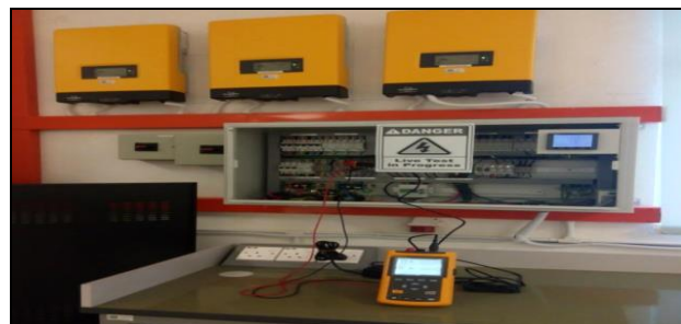
Figure 3: The setup connection of Fluke 43B for measurement and recording data.
