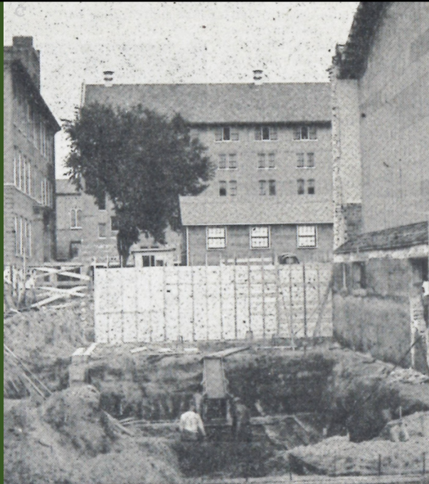
EXCAVATION for the new addition to the gymnasium.
