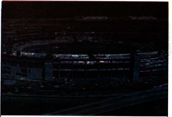
Construction continues on the Cleveland Browns stadium on the shore of Lake Erie. The Browns first season will start in 1999.
