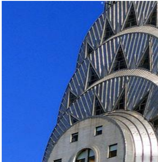
Fig-13, The pinnacle of New York's Chrysler Building is clad with type 302 stainless steel..
