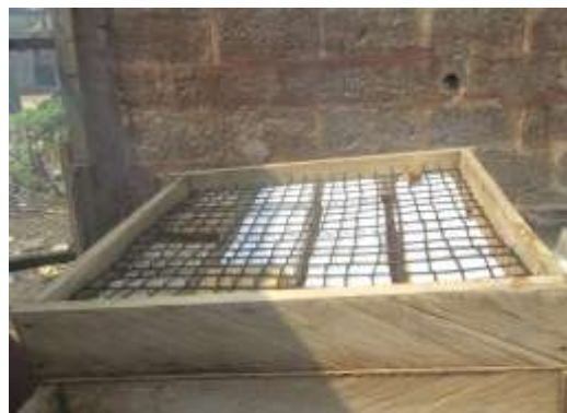
Plate 2: Formwork for polymer rod waffle slab
