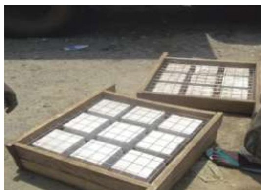
Plate 2: Formwork for polymer rod waffle slab
