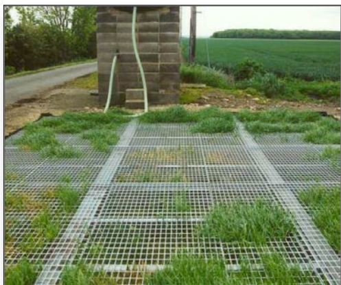
Common design for a biobed. (photo courtesy of: http://www.fwi.co.uk/articles/15/01/2009/113811/integrated-crop-management-cuts-costs-and-benefits-wildlife.htm )
