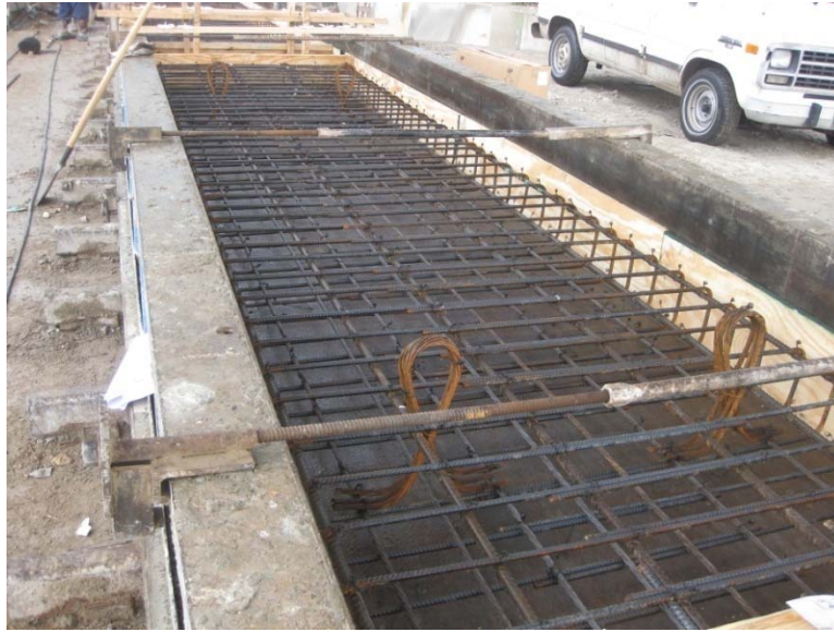
Figure 3.5 Reinforcement Cage for a Typical TPSB
