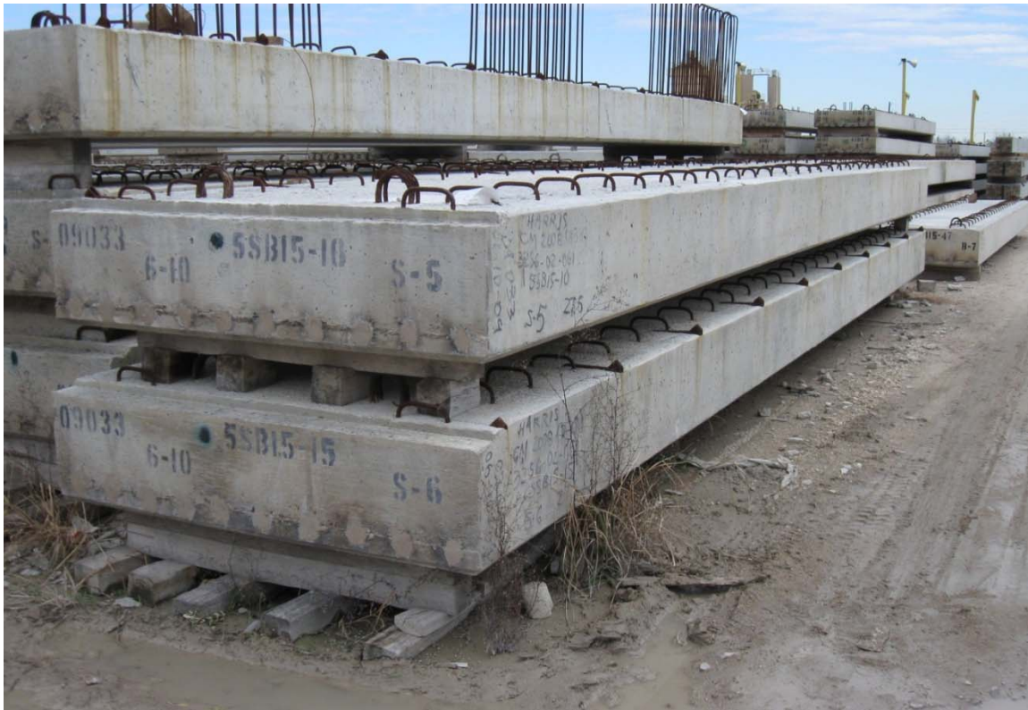
Figure 1.1 Typical Thin Prestressed Slab Beams
