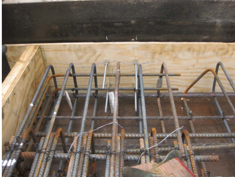
Figure 3.6 3/8 in.-Diameter Threaded Rod and Coupling Nuts Fixed on the Side Formwork
