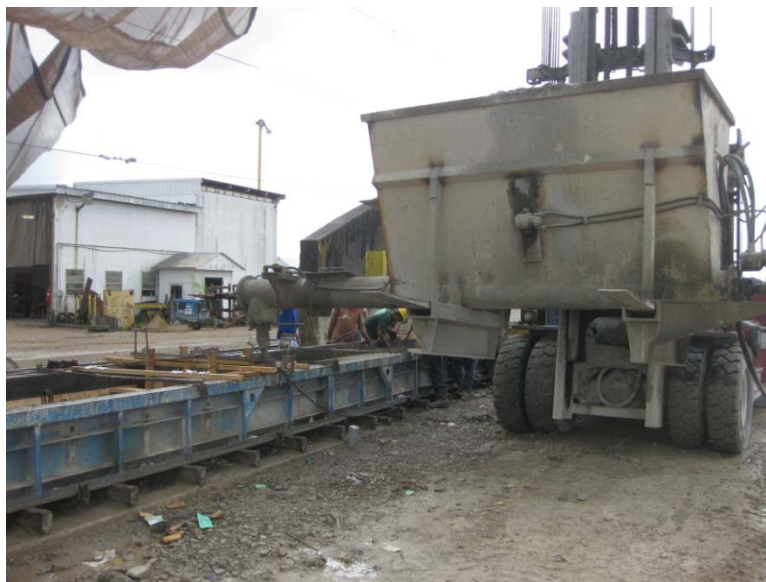
Figure 3.7 Concrete Pouring Using a Mobile Hopper
