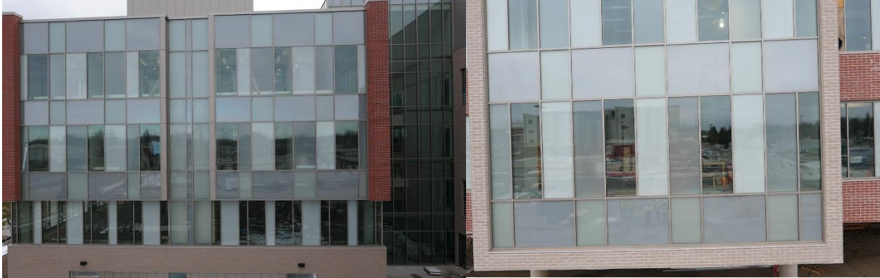
Figure 4.9: Large Lambertian surfaces in the building under inspection
