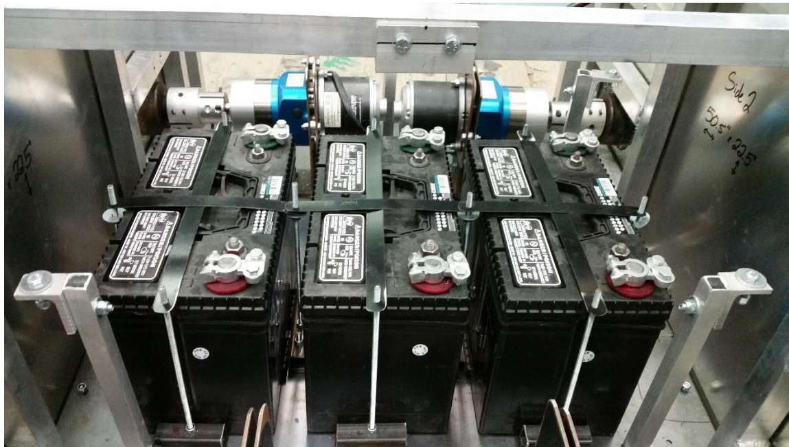
Figure 73 - Batteries Installed in Rover
