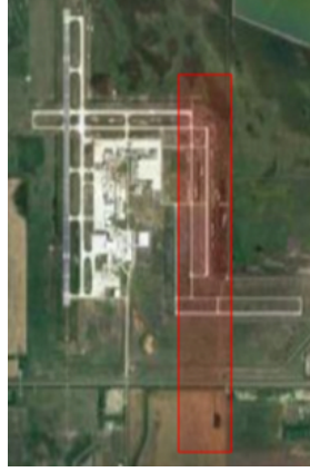
Figure 9: A geometric fence, indicated in red, that was created around the Grand Forks International Airport’s runway 35R.
