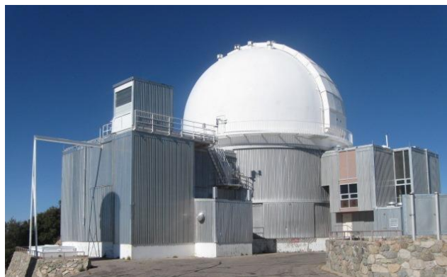
Fig. 16 – NOAO 2.1-meter telescope housing complex at KPNO: The multi-story housing complex of the NOAO 2.1-meter telescope at KPNO (center) and auxiliary 0.9-meter telescope housing (left) which formerly provided the feed for the Coude spectrograph instrument in the lower level of the building.
