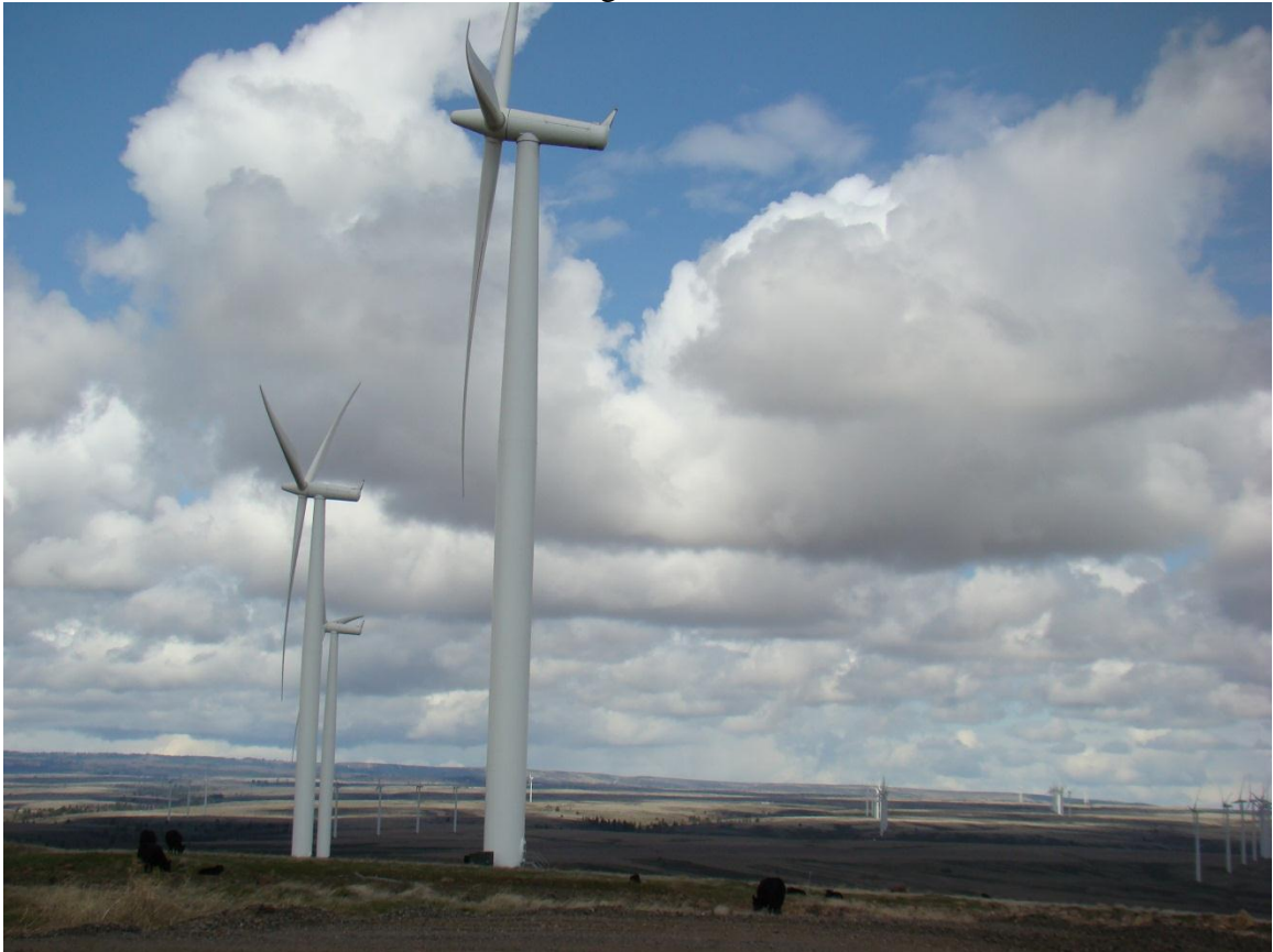
80 meter Siemens 2.3 megawatt wind turbine, White Creek Wind Farm, Roosevelt WA. 2009. Personal photograph by Author. JPEG.
