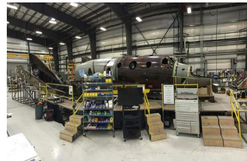
SS2, second vehicle under construction, January 2015
