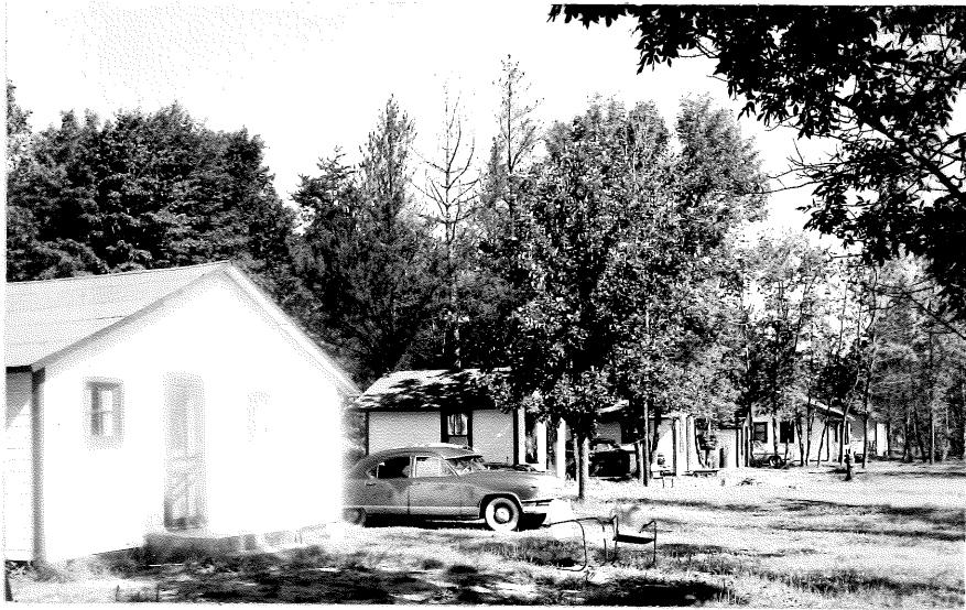
Figure 13. TYPICAL SEMI-MODERN CABINS. (Birch Villa Resort, Cass Lake).
