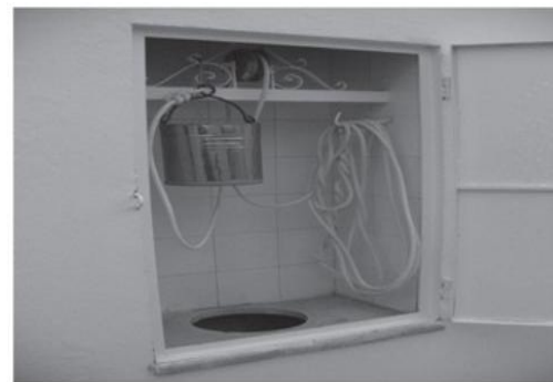
Figure 02: A water harvesting in a depletion of Majel in a modern villa in Tunisia Sfax (Verdeil, 2007)
