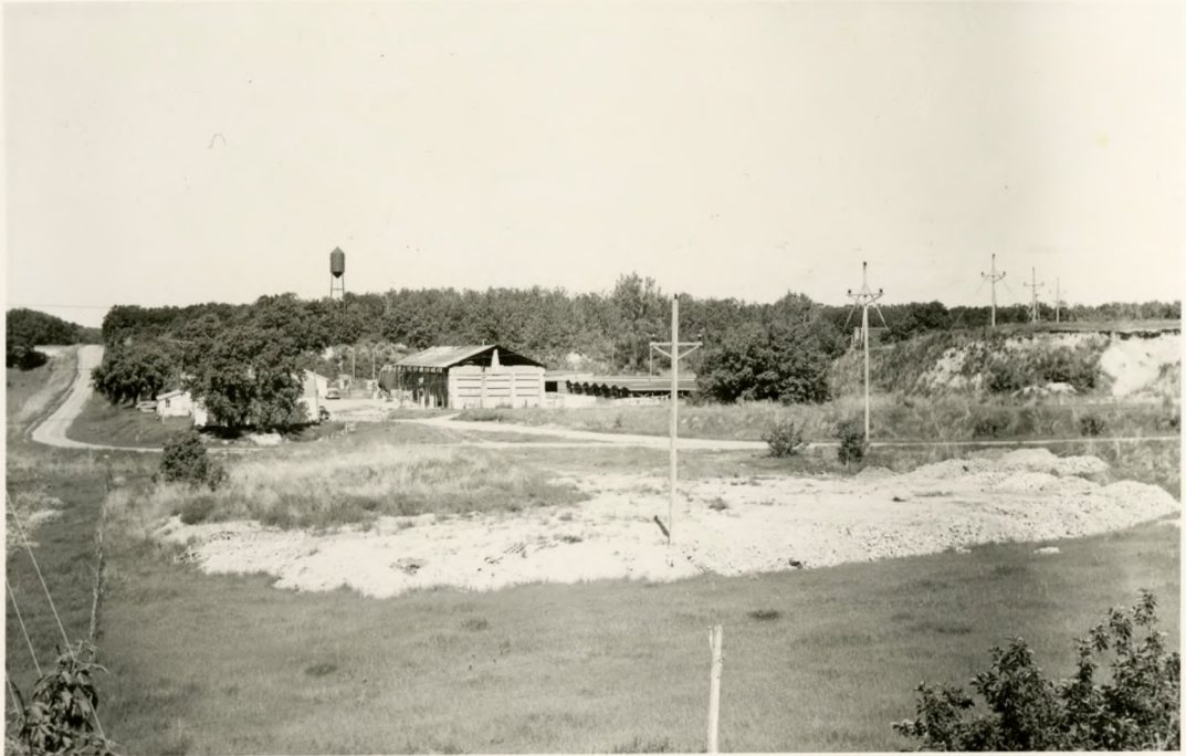
Fig. 16. Red River Valley Brick Company, Fertile, Minnesota. Note the bank of clay on the far right. This marks the farthest northern extent of the Sand Hill Delta. The light material in the foreground is faulty brick that is dumped there for fill.
