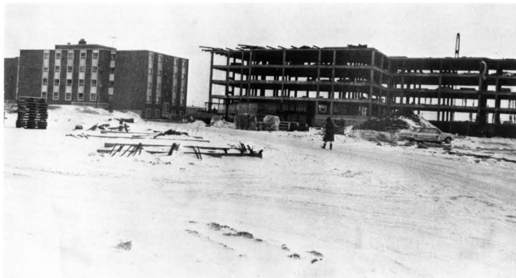
The West residence hall complex under construction, 1967.
