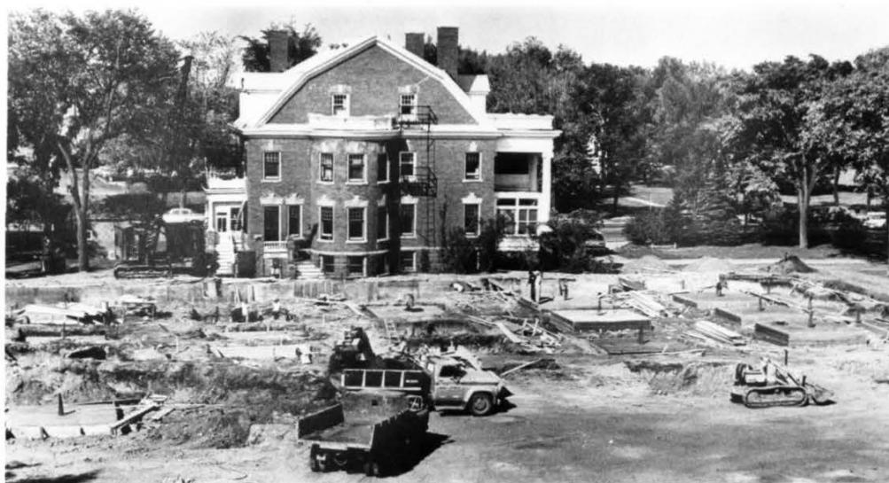
When construction began in 1967 on nearby Gamble Hall, most people assumed that Oxford House, the former president's home, soon would be coming down; instead, a successful drive was begun to save and restore the historic structure.
