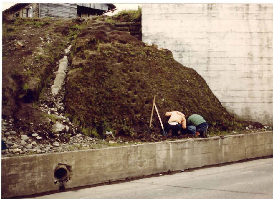
Figure 12. Photograph of the north-facing Puerto Varas Railroad Site roadcut exposure taken from across Calle San Jose. The photograph shows the railroad bridge abutment, concrete retaining wall and lahar deposits, vegetation covered, above the peat. Peat horizon is being examined by Allan Ashworth (left) and Howard Mooers (right).
