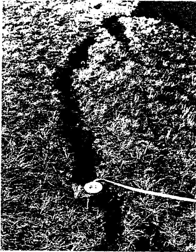
Figure 28. Bank-Parallel Bank-Top Fracture, Lake Sakakawea State Park.
