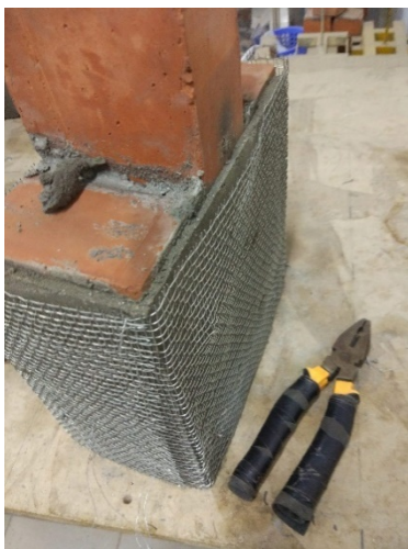
(i) After 1 st layer of plastering
