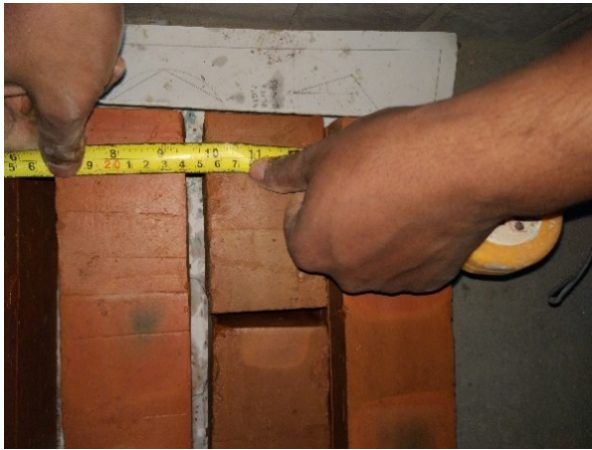
(c) Maintaining 10 mm mortar thickness
