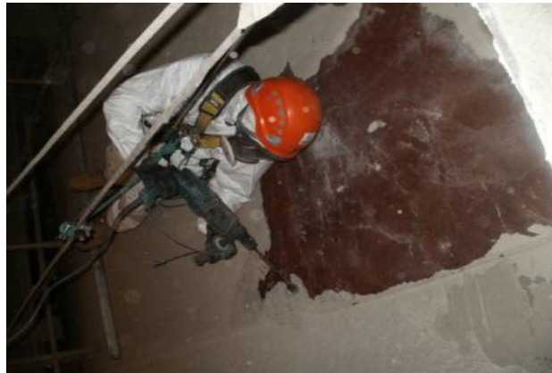
Figure 4: Worker cleaning inside silo using impacting tool
