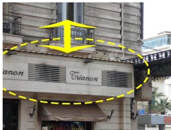
Figure 39: signage compatible with buildings architectural styles.
