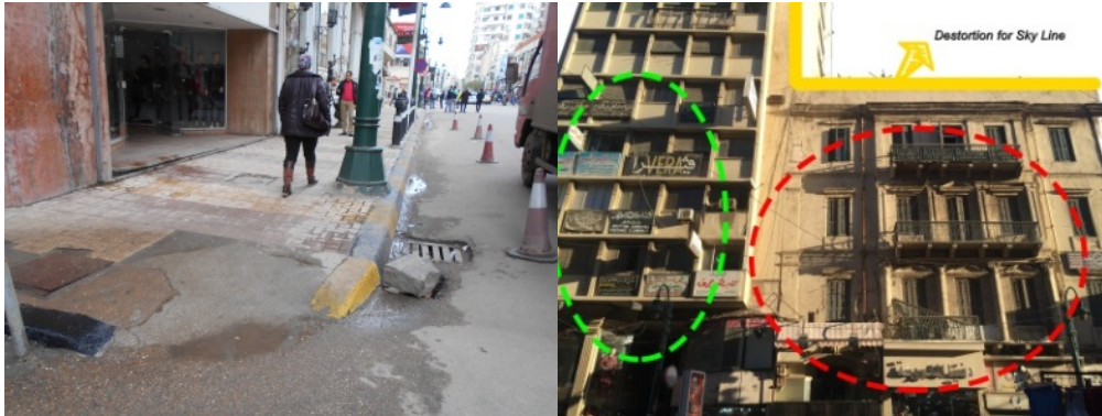
Figure 15: Shows poor finishing material and condition for sidewalks
