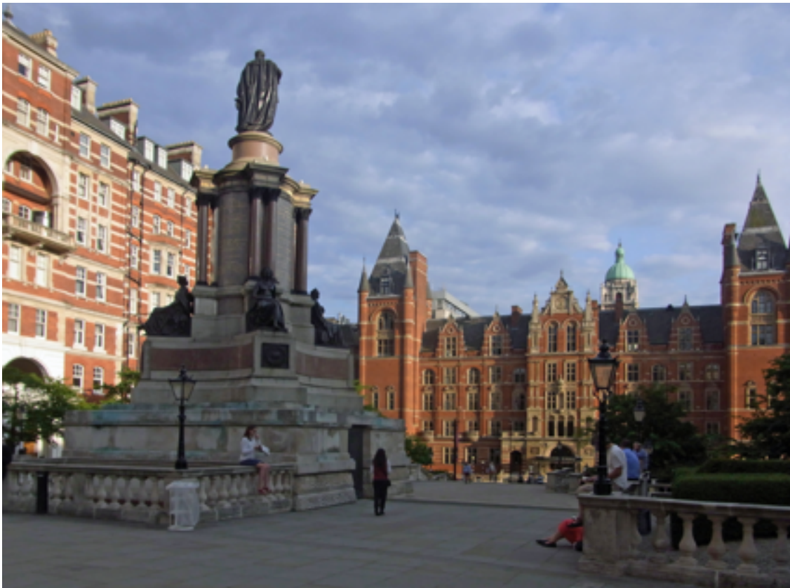
Figure 5.8: View of the site with the Royal College of Music Building and the Albert Court in the background.
