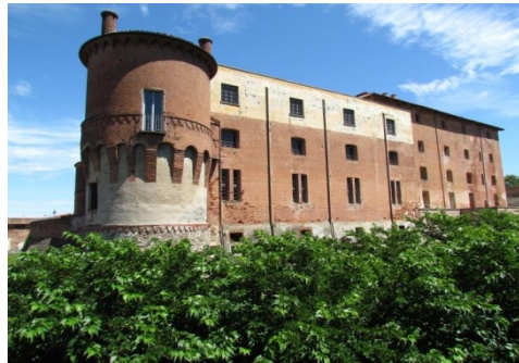
Fig. 1- Saluzzo Castle, view overlooking the hillside
