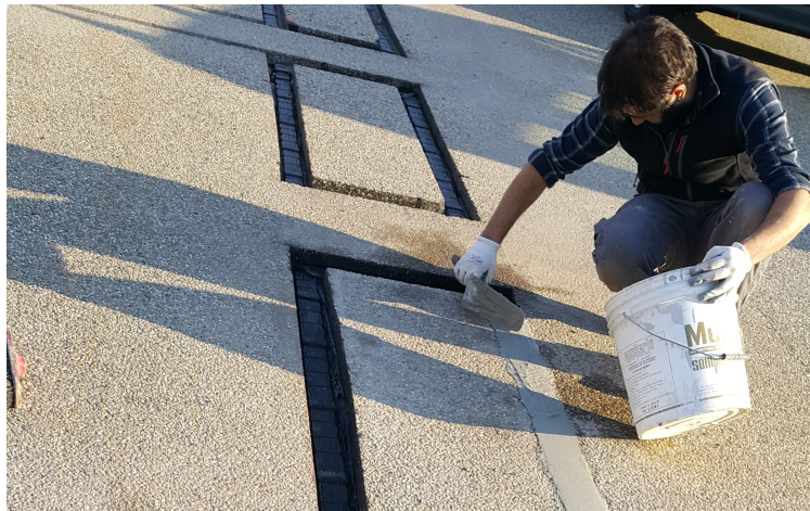
Fig. 5.13: Covering the coil with concrete.
