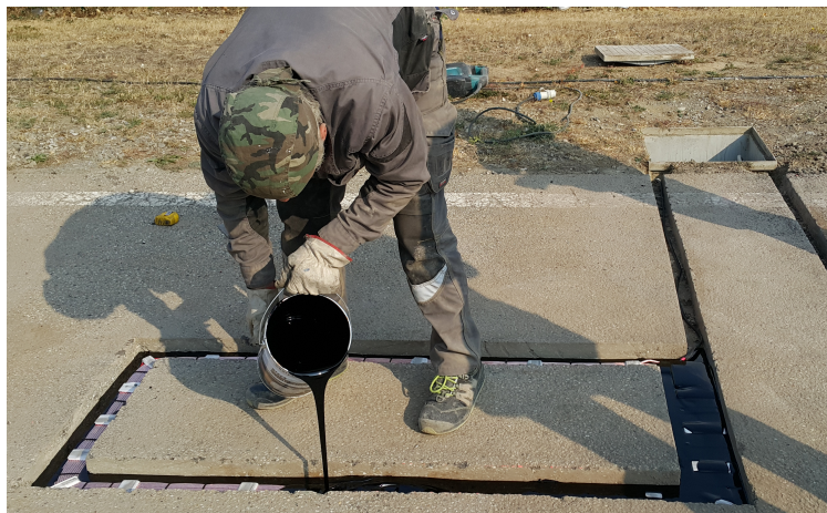
Fig. 5.12: Coating of the coil inside the ground with isolating material.
