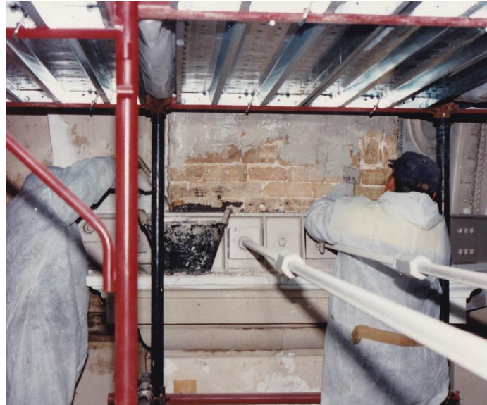
Figure 10. Strengthening work near the insertion of tie rods.
