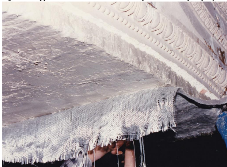
Figure 14. Intrados application of GFRP band for strengthening arch.
