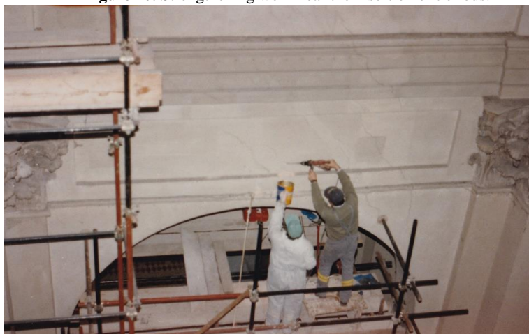
Figure 11. Injections technique for repair of existing cracks.
