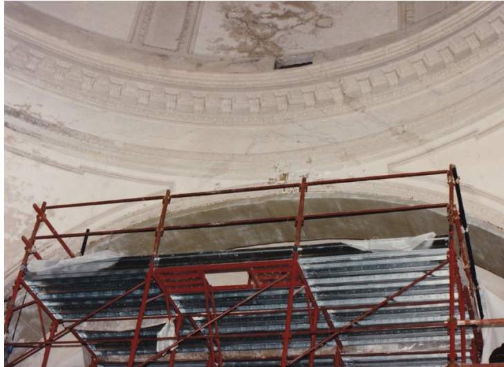
Figure 9. Application of GFRP intrados reinforcement bands on the triumphal arch.
