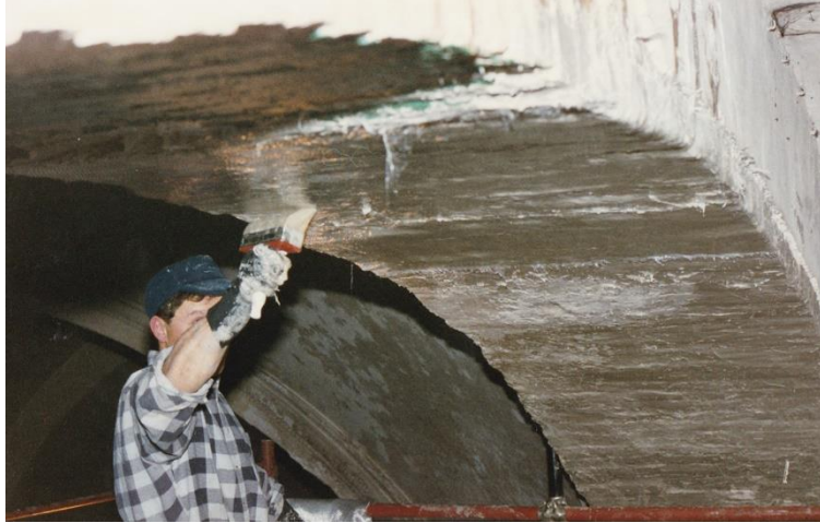
Figure 12. Application on the treated surface of two-component synthetic resin primer in aqueous dispersion.
