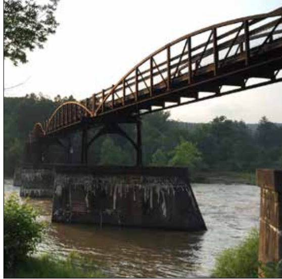
A pedestrian bridge along the 150-mile Great Allegheny Trail.
