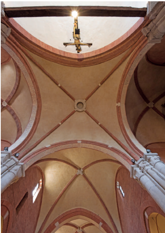
Fig. 10. Rivalta Scrivia Abbey of Santa Maria. Rib vaults covering the intersection between the transept and longitudinal element (photo credit: Marco Gattinoni).
