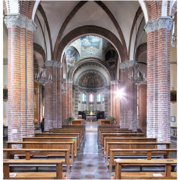
Fig. 5. Vercelli Church of San Bernardo. Interior with rectangular-ribbed vault covering the nave.
