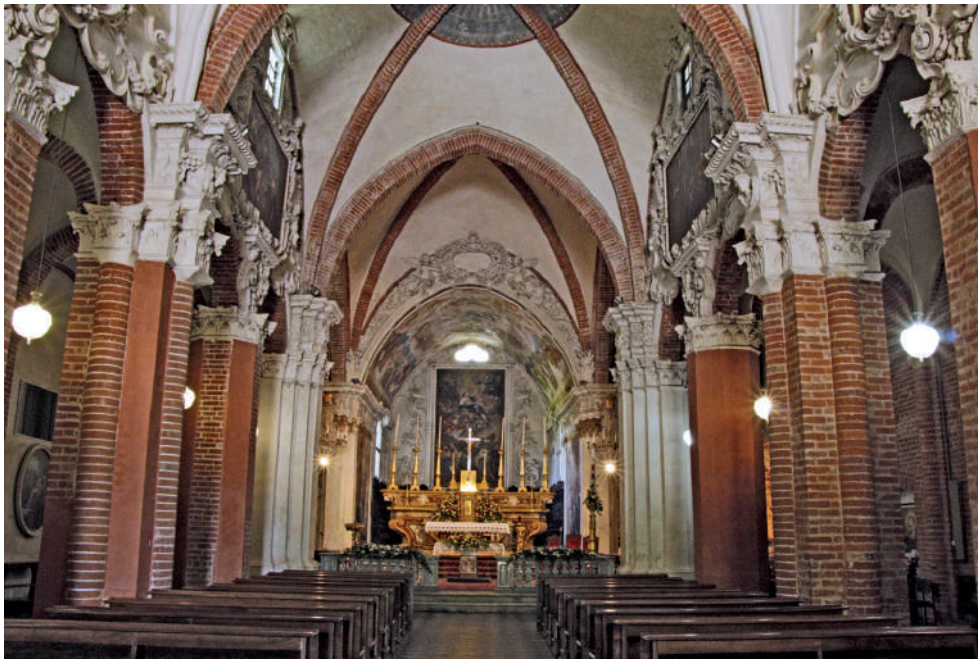
Fig. 7. Casanova (Turin) Abbey of Santa Maria. Interior of the central nave with pointed rectangular and tore rib vaults.
