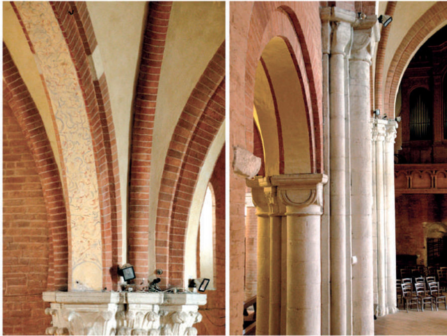
Fig. 11. Rivalta Scrivia Abbey of Santa Maria. Transverse arches and torus-profile rib vaults. Polystyle pillars of the transept aisles.
