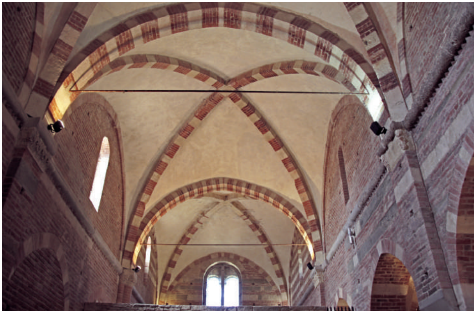
Fig. 14. Vezzolano Abbey of Santa Maria. Ribbed vaulting system in the central nave.
