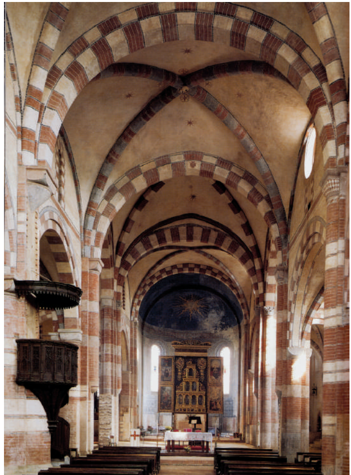
Fig. 6. Staffarda (Cuneo) Abbey of Santa Maria. Longitudinal section of the church with rectangular or torus rib vault.
