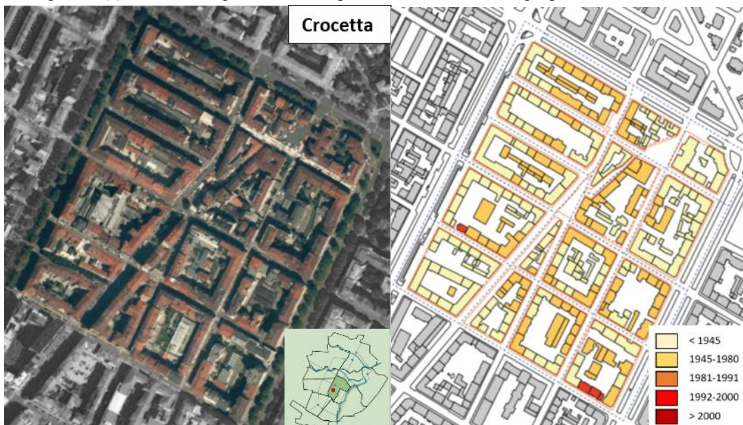
Figure 12(b): Urban configurations of Crocetta district with buildings' period of construction.
