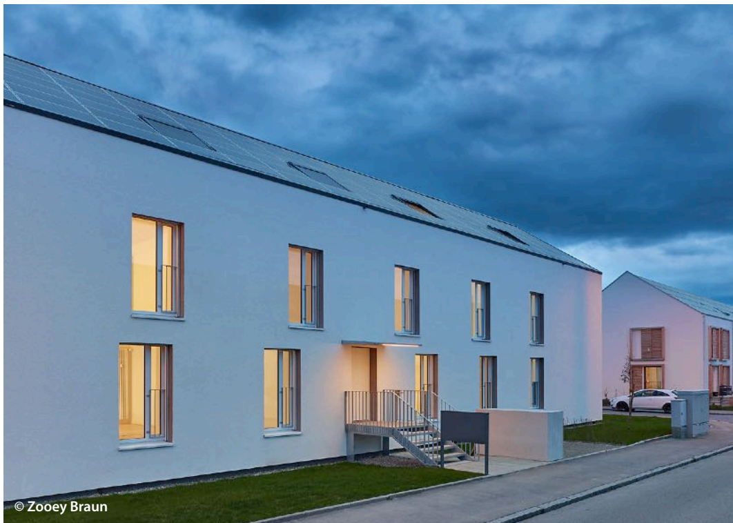
Street view of the south façade after retrofit Building integrated photovoltaic roof, floor-to-ceiling windows and main access
