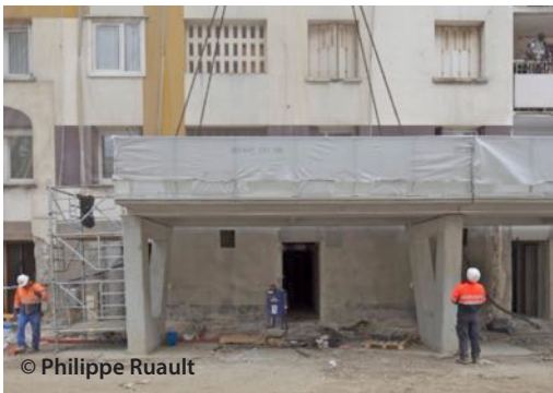
Top: Buildings before retrofit Bottom: Loggias under construction
