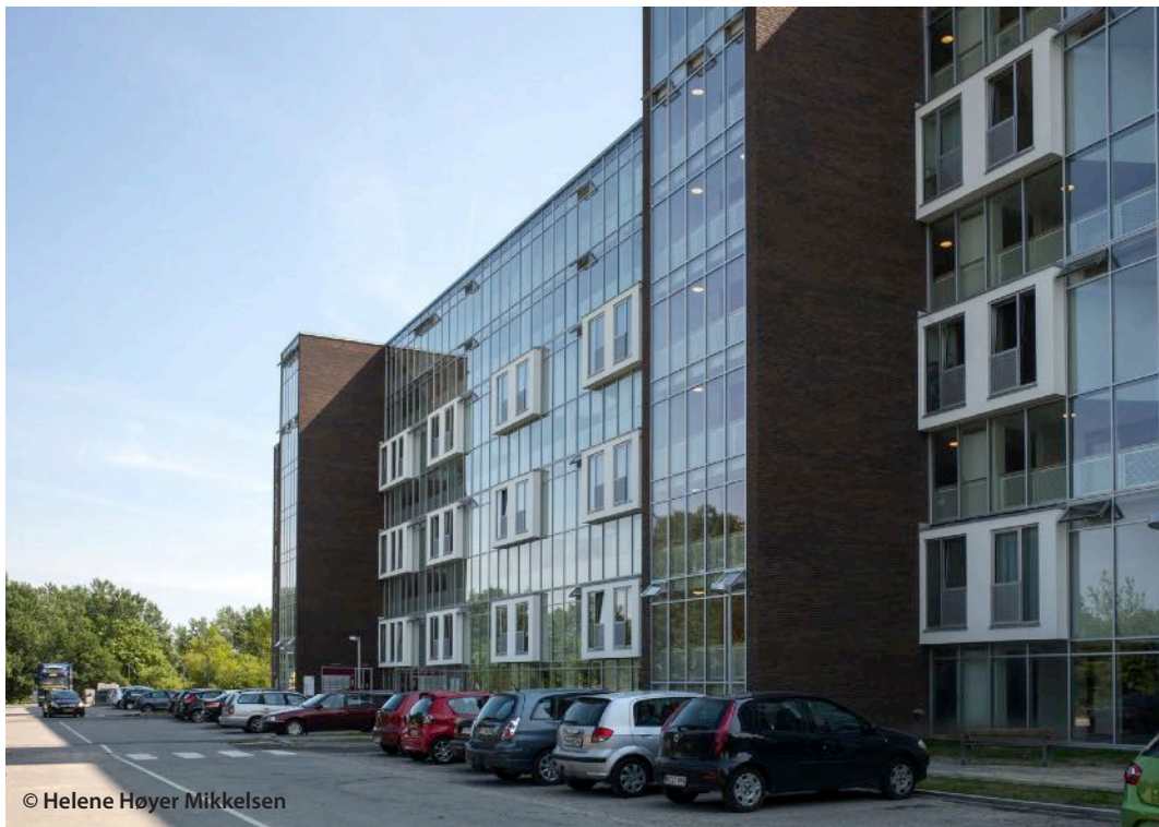
Building after retrofit Exterior of the north façade with added stair and elevator towers
