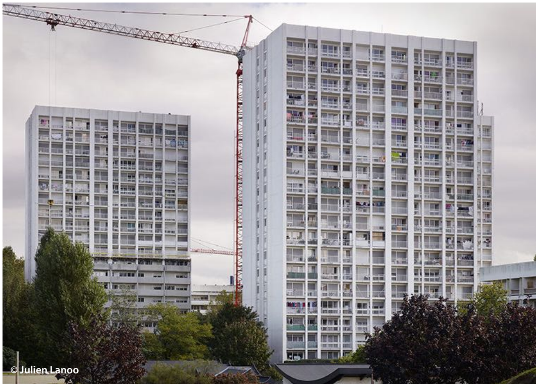
Buildings before retrofit
