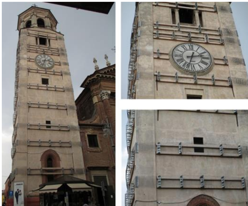
Figure 37: the belfry of the Fossano Cathedral with the strengthening intervention.
