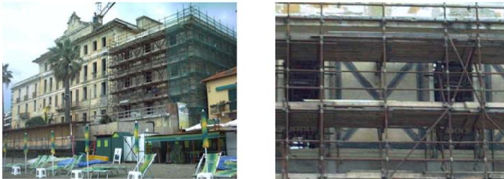
Figure 30: restoration intervention realised on the masonry external façade. Source (Credali, 2009).
