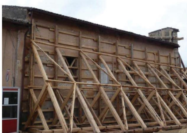
Figure 20: propping intervention of lateral wall of church of Onna (AQ). Source (Modena, et al., 2011).
