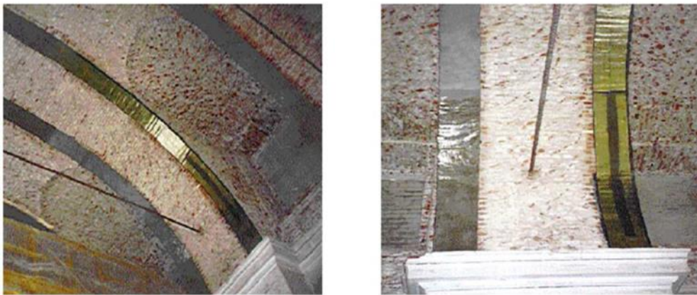
Figure 34: Complesso di Venaria Reale (TO) – Strengthening intervention with strips placed to the intrados and extrados of the vaults. Source (Credali, 2002).
