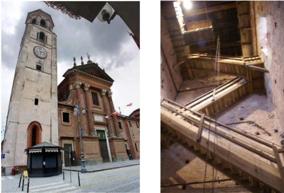
Figure 36: the Fossano belfry; wood ramps located inside the tower.
